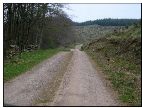
Photo 1: View Looking East Showing Vertical Alignment
