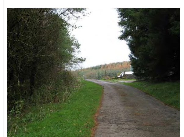
Plate 10: Looking North Towards High Auldgirth
