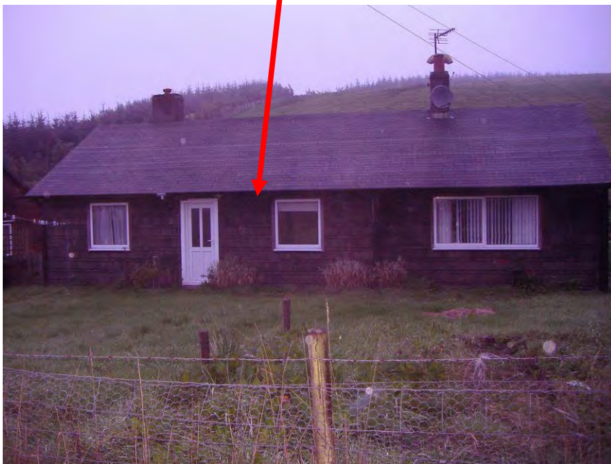
Photograph 3 – 29.09.2011 - One Soprano pipistrelle emerged from above the wall head to the right (east) of the door on the rear (south-facing) side of No. 2.
