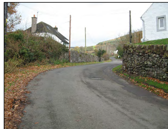
Photo 3: View looking North East at Auldgirth Inn
