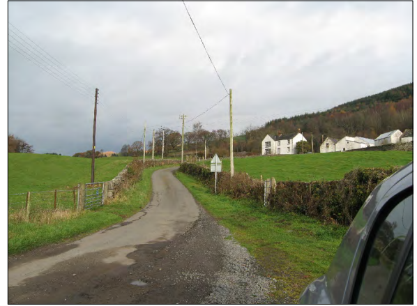
Photo 1: View Looking North East Towards Start Point of Proposed New Access Track
