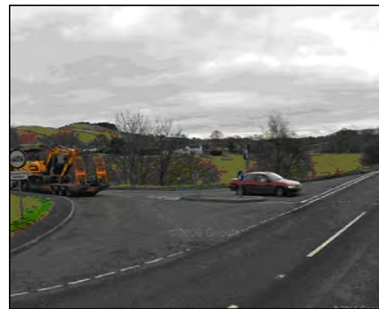
Photo 1: View looking at Auldgirth Junction on A76
