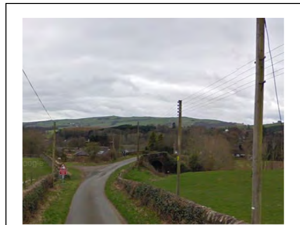
Plate 7: Looking South Towards Existing Railway Bridge
